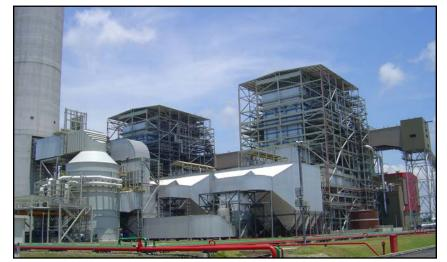
Environmental equipment at the Tanjung Jati power plant includes low  $NO_x$  burners, wet FGD system, and electrostatic precipitators.
