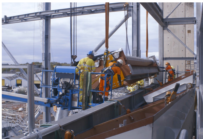
One of the ten modular DynaGrate sections being lifted into place.
