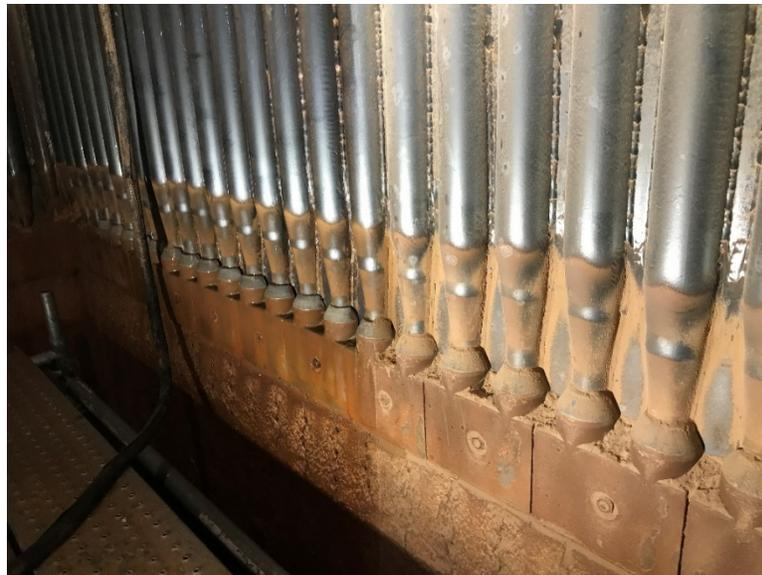
**Figure 10.** Lower Furnace Refractory and RDZ Zone After Several Years of Operation (note that the shine on the tubes was for UT measurement during the outage; it was not from erosion)
