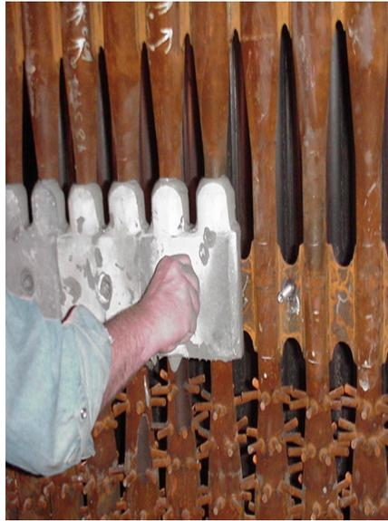
**Figure 9.** Initial Installation of RDZ on New CFB Steam Generator
