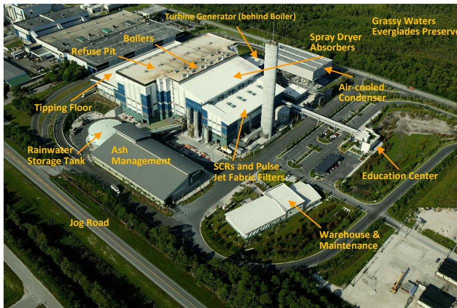
**Fig. 4** PBREF No. 2 plant overview (from June 2015 looking from northeast to southwest).
